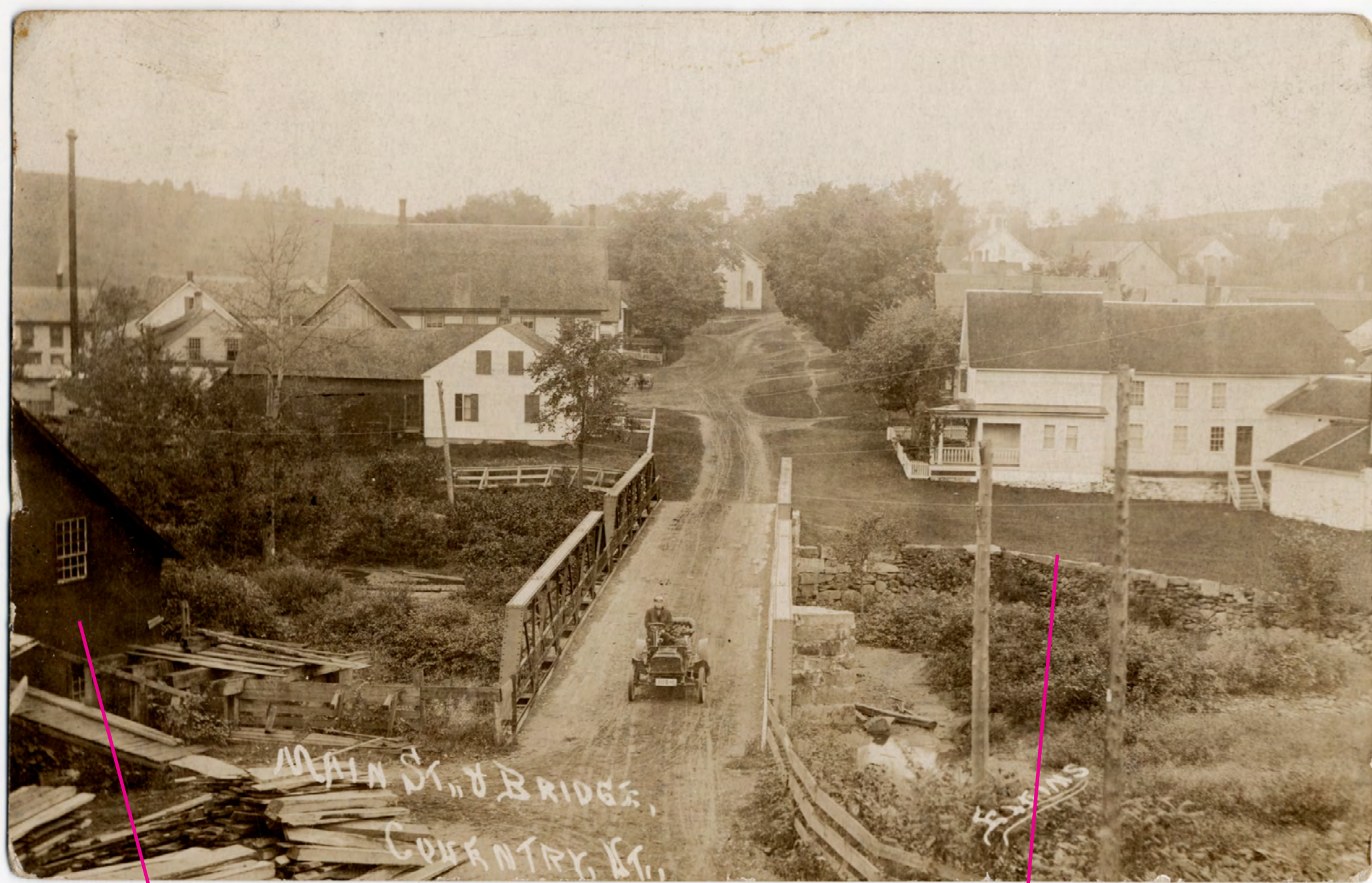
Early Rte 14 steel bridge across Black River, Coventry, circa 1910
