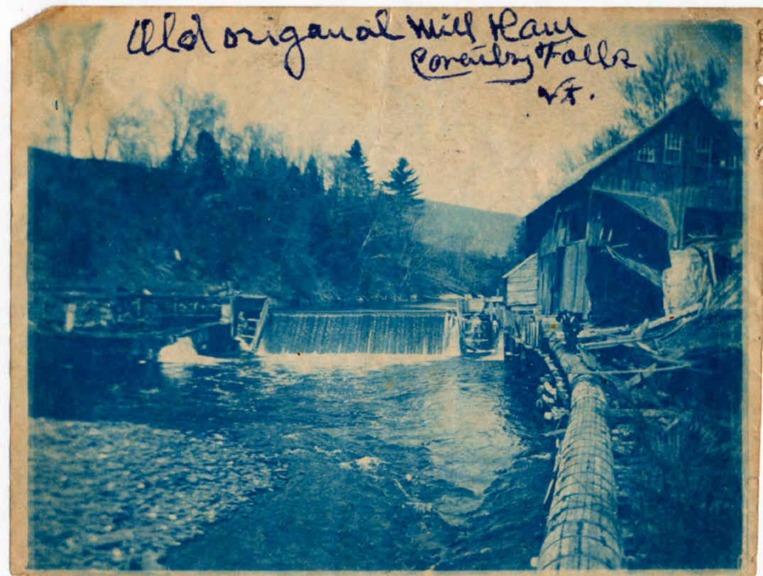
Mill district - Black River, circa 1890, starch factory on right. Penstock provided water to power bobbin mill downstream Grist mill in picture below to left of this picture.
