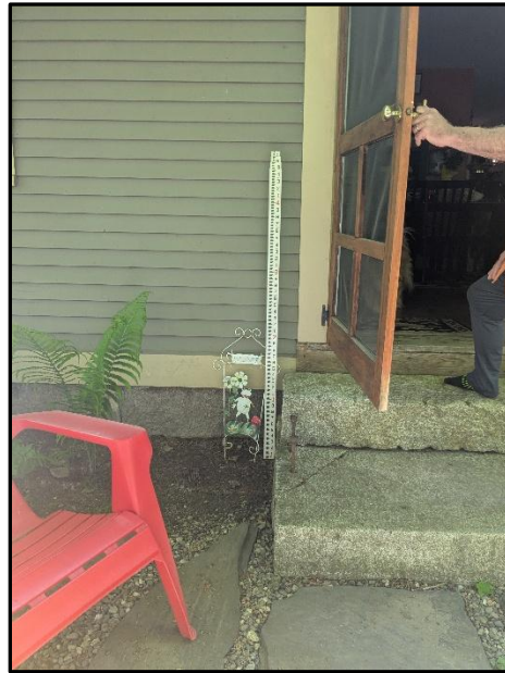
Photo 8a and 8b. The front of the home at 36 Conway Court. The owner noted that ice and water have reached the sill of the doorway (approximately 2 ft above the adjacent ground) but haven't overtopped into the home.
