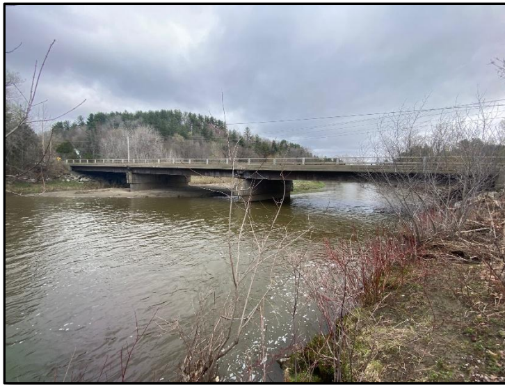
Photo 3. Looking at the Rte 105 Bridge from upstream to downstream
