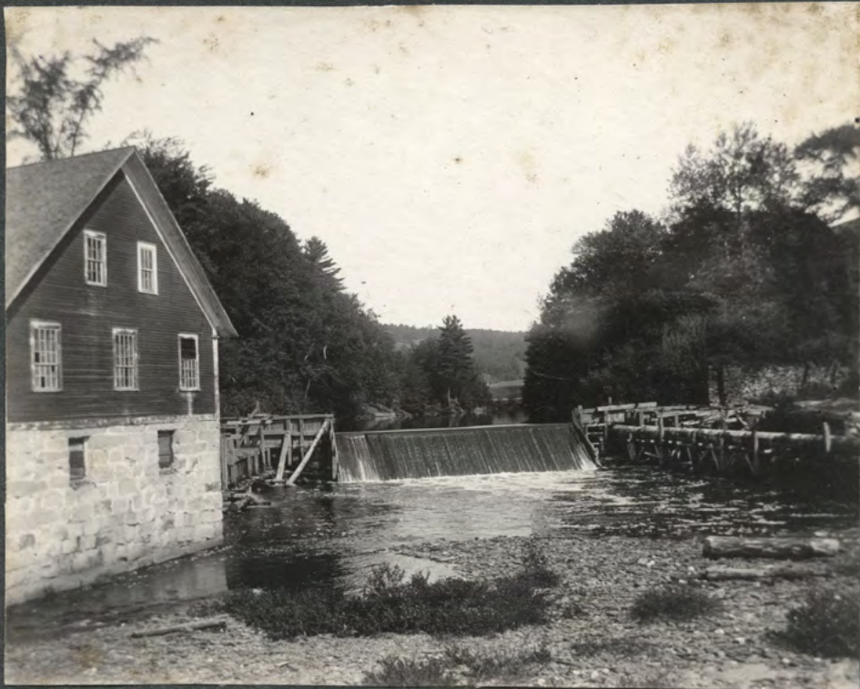
Grist mill, mill dam and penstock, Black river, Coventry village, circa 1900. There were mill dams like this upstream - in Irasburg, Albany, Craftsbury - all helped to deter ice jams by trapping ice during thaws at varying points along the river.
