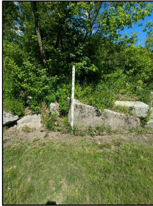
Photo 5. Large riprap along the right bank just upstream of the Rte 105 bridge. The riprap was placed along the right bank when the bridge was constructed (see Photo 2a.)
