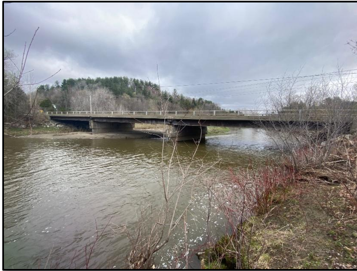
Photo 3. Looking at the Rte 105 Bridge from upstream to downstream
