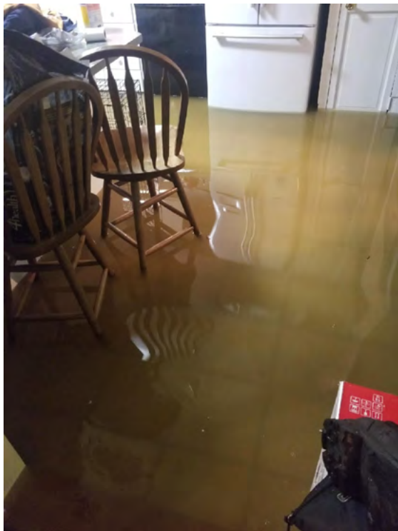
Hardwood kitchen floor, dry wall, insulation, furniture, personal items destroyed
