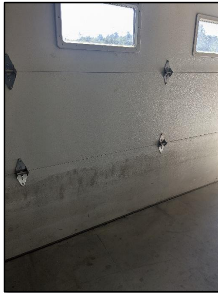
Photo 9a and 9b. The recently raised garage at 88 Main St (left). Sediment line inside the garage door (right). This is a remnant from the July 2023 open-water flood event.
