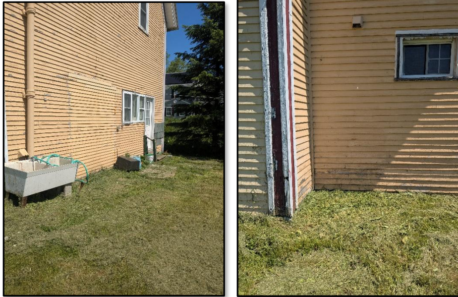
Photo 11a and 11b. The entrance to the lower apartment at 235 Main Street (left). Sediment and damage to siding from the July 2023 flood were observed on the south side of 235 Main Street (right).
