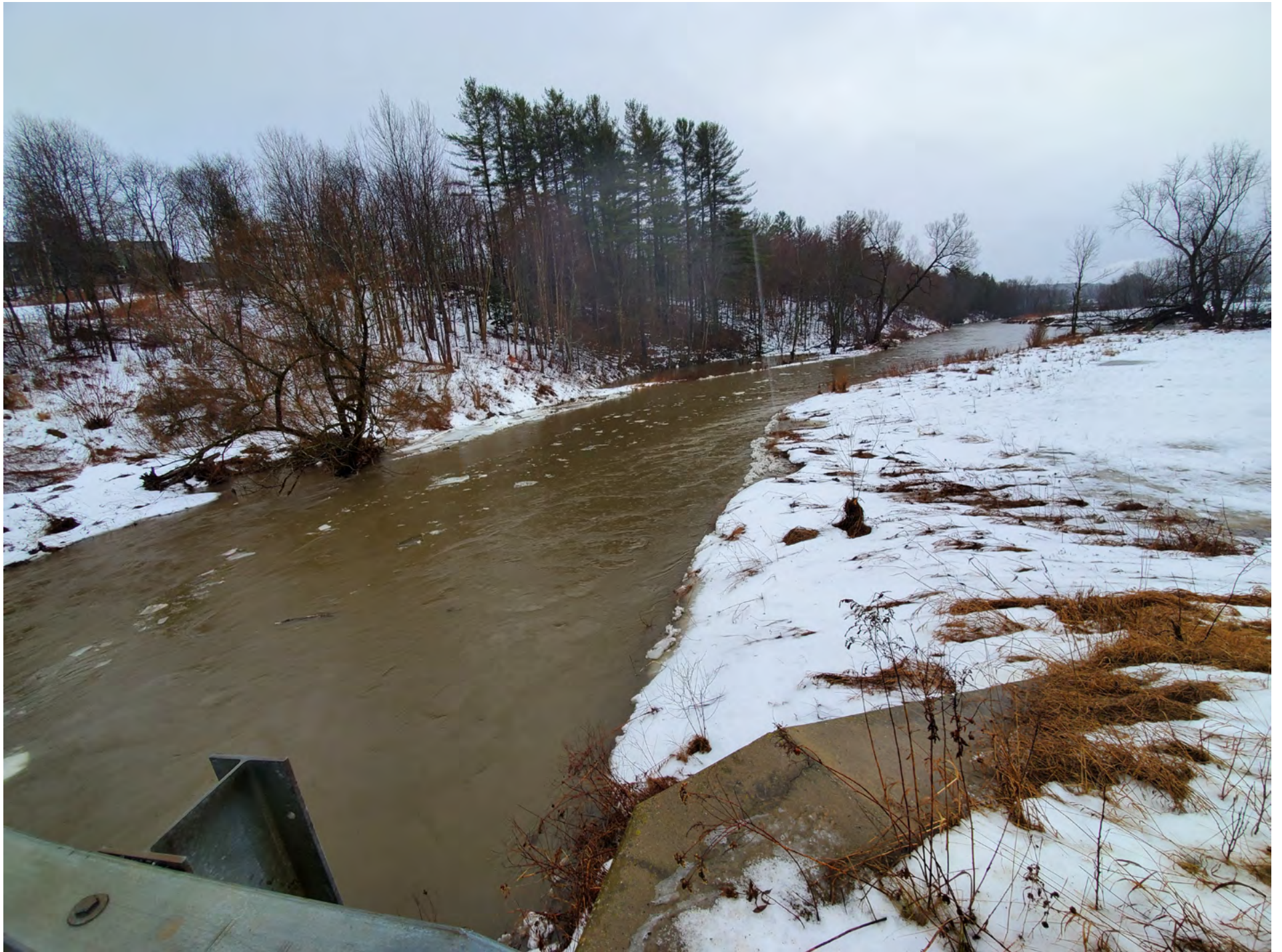
Ice jam and high water Jan 12, 2020 - At bridge above Upper Falls
