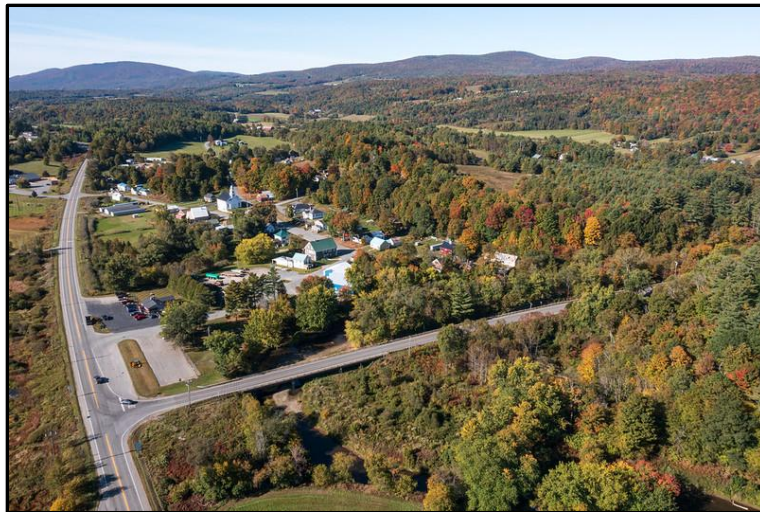
Photo 1. Overview looking south of the Town of Coventry and the intersection of Rte 5 (N-S) and Rte 105 (E-W)
