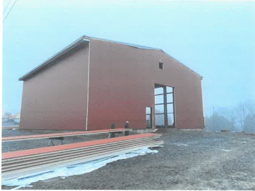
Leachate Pre-Treatment System Building
